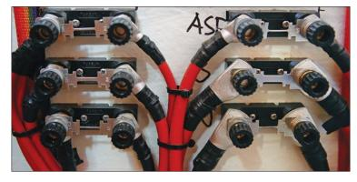
accidental short circuits. Note that there are still exposed conducting surfaces between the fuses. **Bottom right**—These hand-tightened knurled knobs are convenient for rapid fuse changes without tools but do not create adequate pressure for high-current circuits. Bolted connections are needed.
