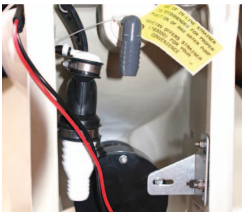
The guts of the toilet were simple enough, with the macerator pump under the bowl
