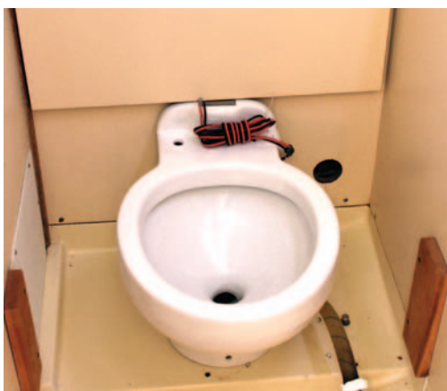
Dry-fit the toilet first to get an idea of hose and electrical cable runs
