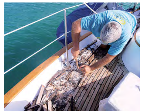
The farthest outboard teak planks were set in a white bedding compound and came up quite easily, at left. As [redacted] worked his way inboard, he found a tar-like compound that was much stickier, center. The teak from then on broke off in smaller pieces, at right.
