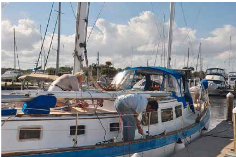
...so [redacted] had to cut the mast at deck level. One of the necessary jobs when changing a rig is the repositioning of chainplates
