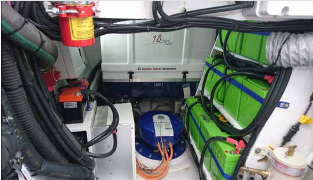
This neat OceanVolt serial hybrid installation includes a large bank of lithium-ion batteries at right and a Fischer-Panda generator in a box at center rear.
